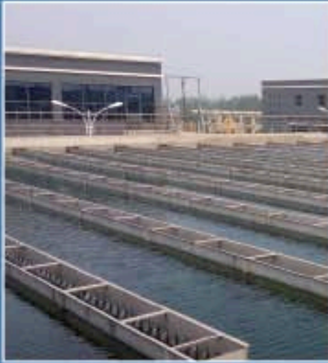
MUNICIPAL DRINKING AND WASTEWATER DISINFECTION
